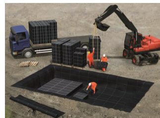
Figure 7: Positioning the infiltration ditch elements
