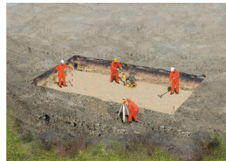
Figure 5: Preparation of the levelled ground
