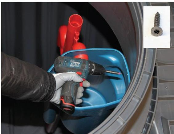
Secure sampling tank to tank dome with Spax screw.
