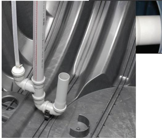
Push sludge return into retaining clip and additionally secure with Spax screw. At the top of the tank, push the sludge return into the sludge return pipe.
