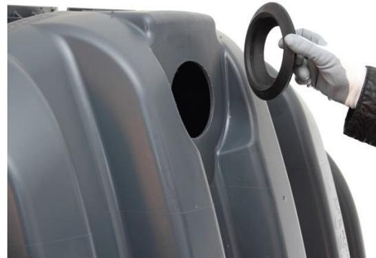
Deburr hole. Insert DN 110 edge seal. The feed-through direction can be seen in the previous diagram.
