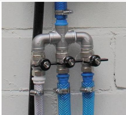
The aeration hoses are connected to the two 3/4" hose connectors. The sludge return hose is connected to the 1/2" connection.
