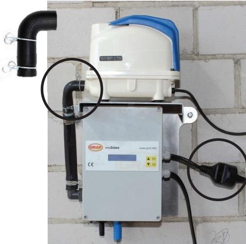
The compressor is placed on top of the control unit. Use the rubber bracket for the air connection. The compressor's connector is plugged into the socket on the control unit.
