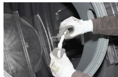
Connect air hose (13mm) to lifter for clear water extraction. Connect air hose (13mm) to lifter for sludge return.
