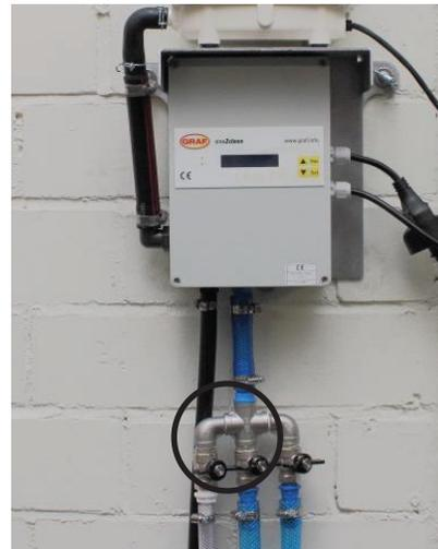
The hose for clear water extraction (1/2") is directly connected to the black hose connector on the control unit. The additional air distributor is connected to the control unit's blue hose connector (3/4").
