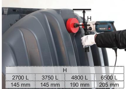
Drill the inflow and outflow with a DN 110 core drill (with a diameter of 124 mm).
