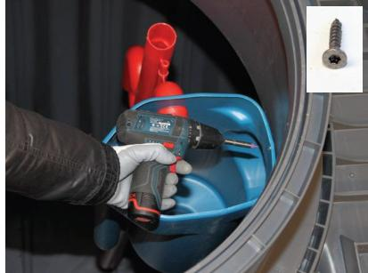
Secure the sampling tank to the tank dome with a Spax screw.
