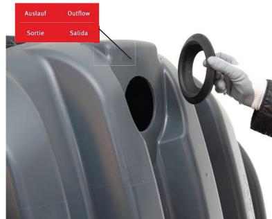
De-burr the hole. Insert the DN 110 lip seal. In the case of the outflow, the direction of the feed-through must be from the inside out. Affix the "Outflow" sticker.
