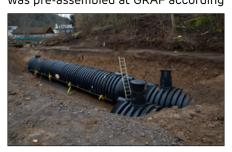
to the project specifications and delivered ready for connection with all accessories as specified in the standard DIN 14230. In addition to a holder for a sign indicating the extraction point, the scope of delivery includes two welded-in plastic suction pipes DN 125, a stainless steel strainer with anti-vortex plate, a firefighting water suction connection with a dipstick and an A-type solid fire hose coupling (110 mm diameter)
