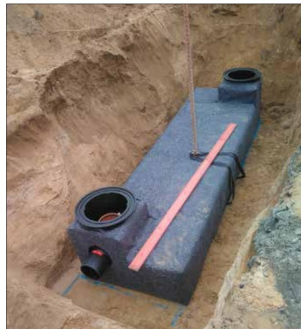
Vario 800 EcoBloc-Sedimentationstank 5880 l
