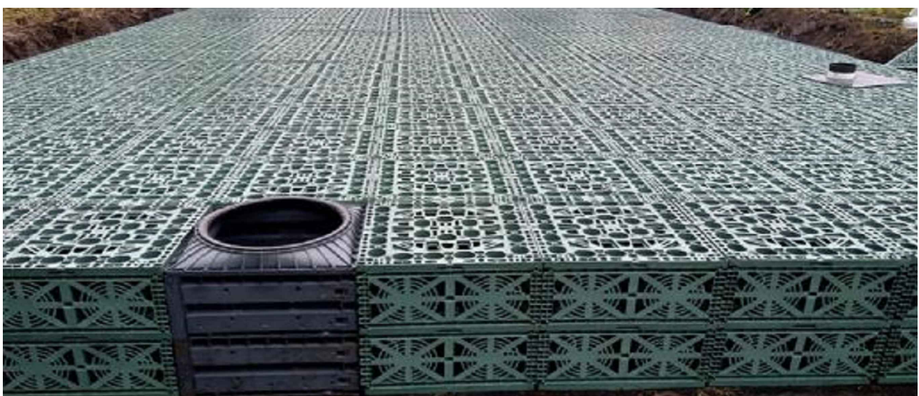
Image shown is of an EcoBloc Light Infiltration Tank with a row of EcoBloc Flex for Inspection / maintenance
