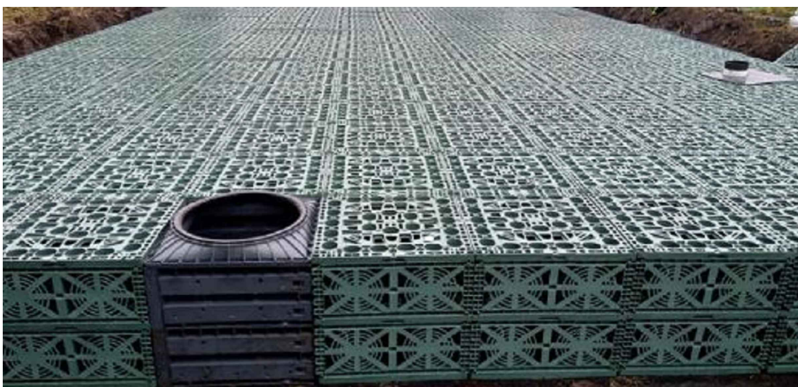
Image shown is of an EcoBloc Light Attenuation Tank with a Vario shaft and a row of EcoBloc Flex for inspection / maintenance
