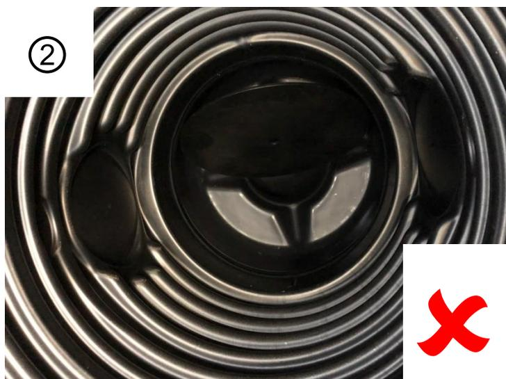
After removing the blockage or the orifice, it must be ensured again that the orifice lies level and horizontally in the vortex flow control shaft body.
